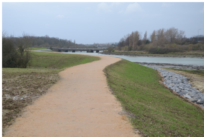
Earlier flood defence work at Portcreek
